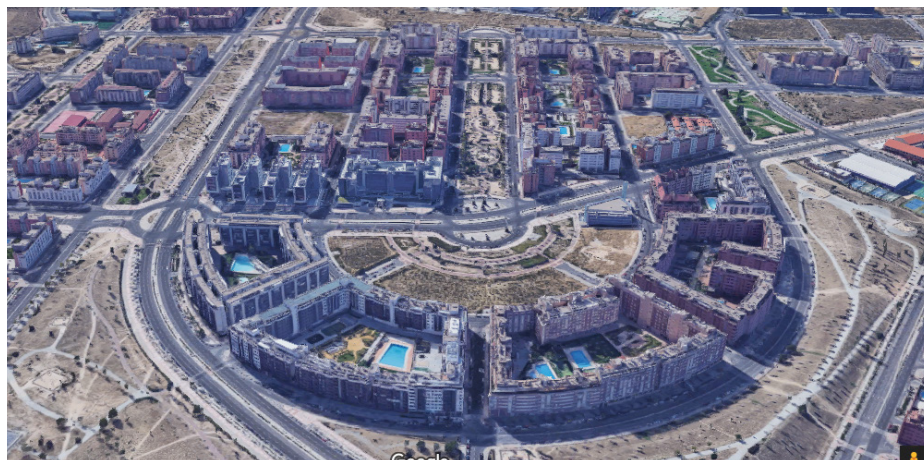
Figure 6.4 | The inner courtyards of Las Tablas gated condominiums. Source: Google Maps. Accessed fall 2018.
